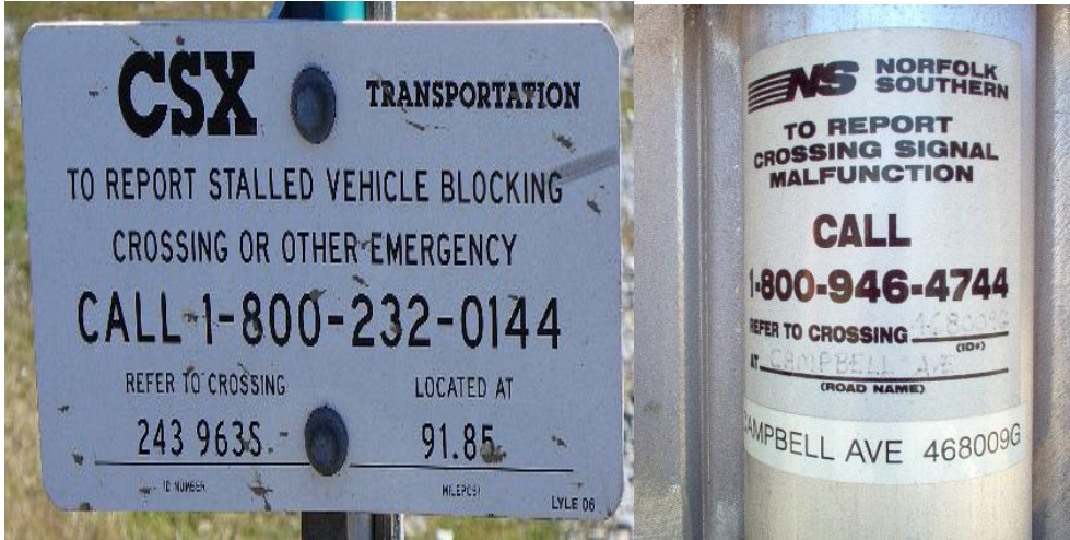
Road crossing number markers
