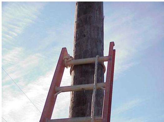
**Step 3:** Flip the rope over the top of the leg so it rests on the top rung.
