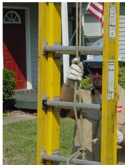
In situations where only one person will be carrying the ladder and no difficulty in maneuvering is likely, the “High Shoulder Method” should be used. As the mechanic has done in Fig. 8, face the foot of the ladder and place one arm between the beams at the balance point so that the ladder hangs under your shoulder.
