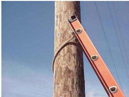
**Step 2:** Wrap the rope around the pole.
